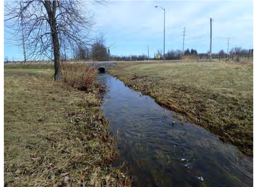
Photo 26. C18 – Atchison Road – Close view of the channel downstream of the culvert outlet. April 11, 2022
