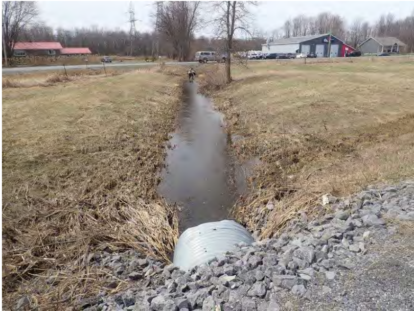
Photo 13. Culvert 17 (C17) – Power Dam Drive – Overview of the culvert inlet and upstream channel. April 11, 2022
