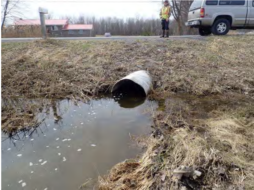
Photo 25. C18 – Atchison Road – View of the culvert outlet. April 11, 2022
