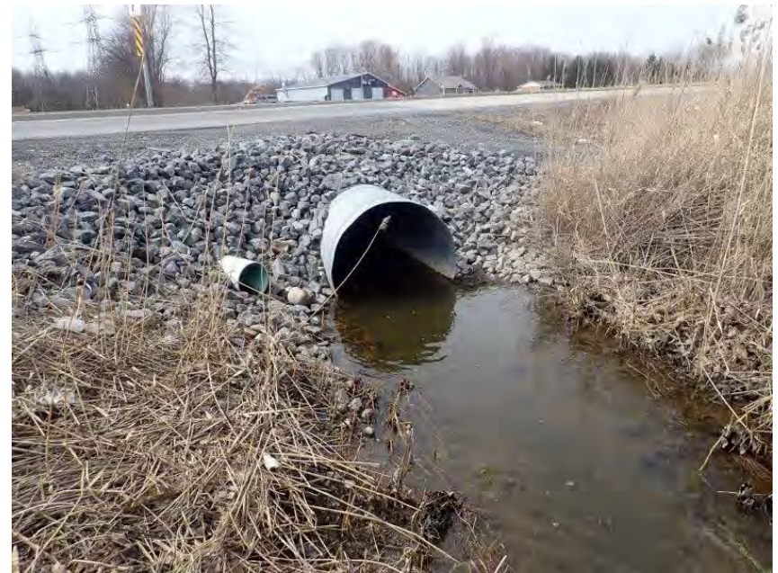
Photo 16. C17 – Power Dam Drive – View of the culvert outlet. April 11, 2022
