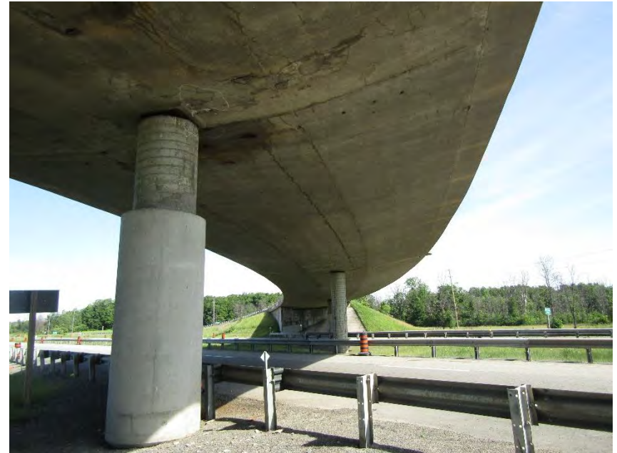
Photo 10. Power Dam Drive overpass – no Barn Swallow nests. June 15, 2022.
