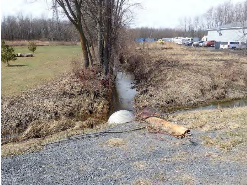
Photo 21. Culvert 18 (C18) – Atchison Road – Overview of the culvert inlet and upstream channel. April 11, 2022
