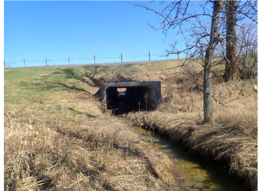
Photo 6. C2 – Highway 401 – View of the downstream channel looking at the culvert outlet. April 11, 2022
