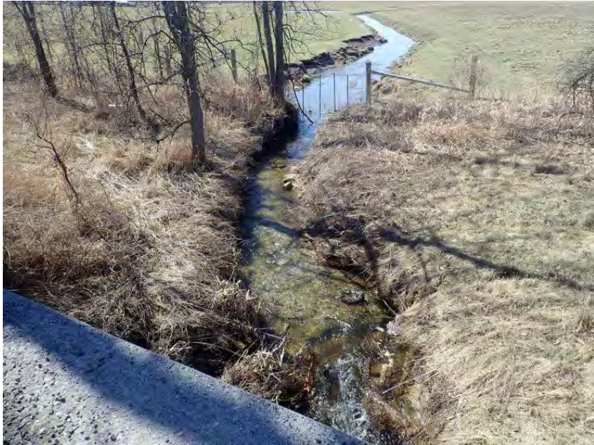
Photo 5. C2 – Highway 401 – Overview of the culvert outlet and downstream channel. April 11, 2022
