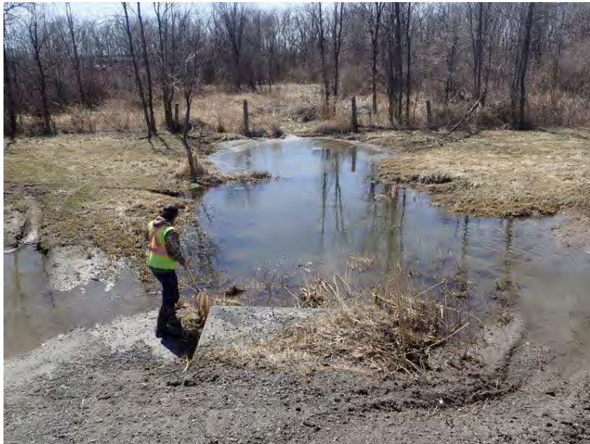
Photo 41. C25 – Highway 401 – Overview of the culvert outlet and downstream area. April 11, 2022
