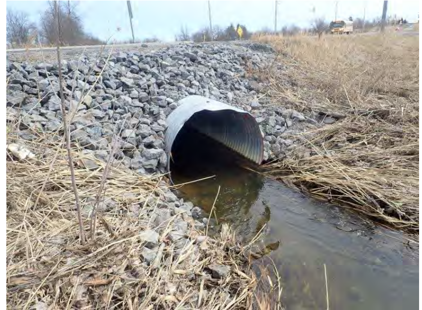
Photo 14. C17 – Power Dam Drive – View of the culvert inlet. April 11, 2022
