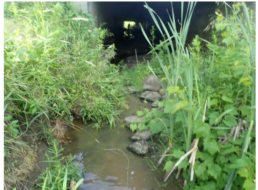
Photo 12. C2 – Highway 401 – View of the downstream channel at culvert outlet during summer. June 29, 2022
