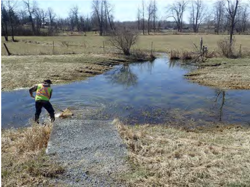
Photo 29. Culvert 22 (C22) – Highway 401 – View of the outlet and downstream channel area. April 11, 2022
