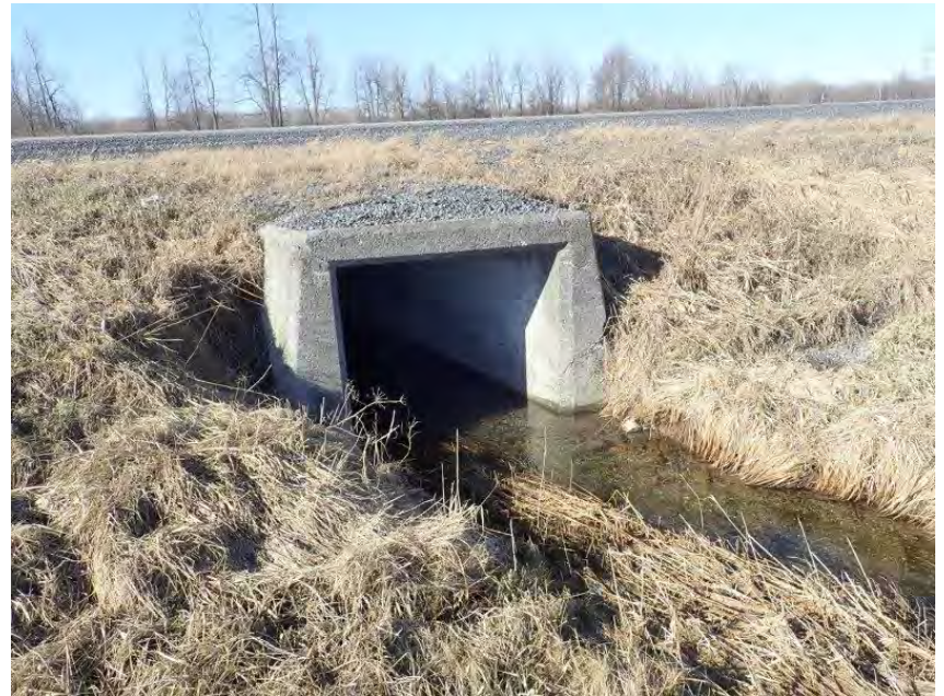
Photo 34. C23 – Highway 401 – View looking at the culvert inlet from upstream channel. April 11, 2022
