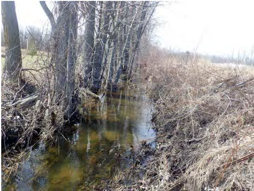
Photo 23. C18 – Atchison Road – Close view of the channel upstream of the culvert inlet. April 11, 2022
