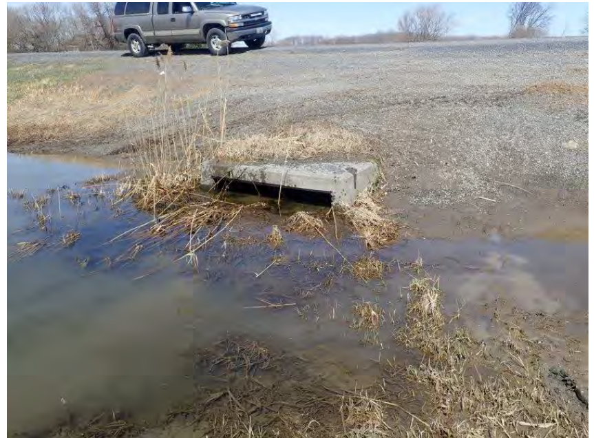
Photo 42. C25 – Highway 401 – View of culvert outlet, downstream area and standing water in ditchline. April 11, 2022
