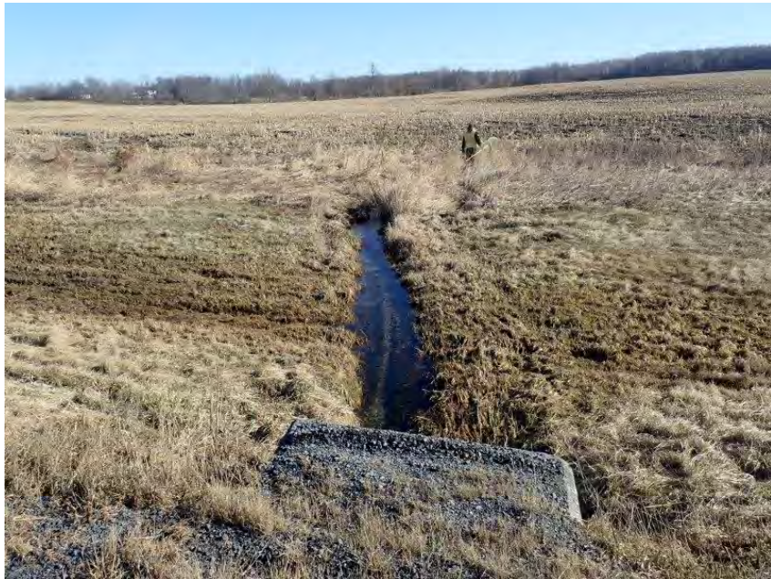
Photo 33. Culvert 23 (C23) – Highway 401 – Overview of the culvert inlet and upstream channel. April 11, 2022
