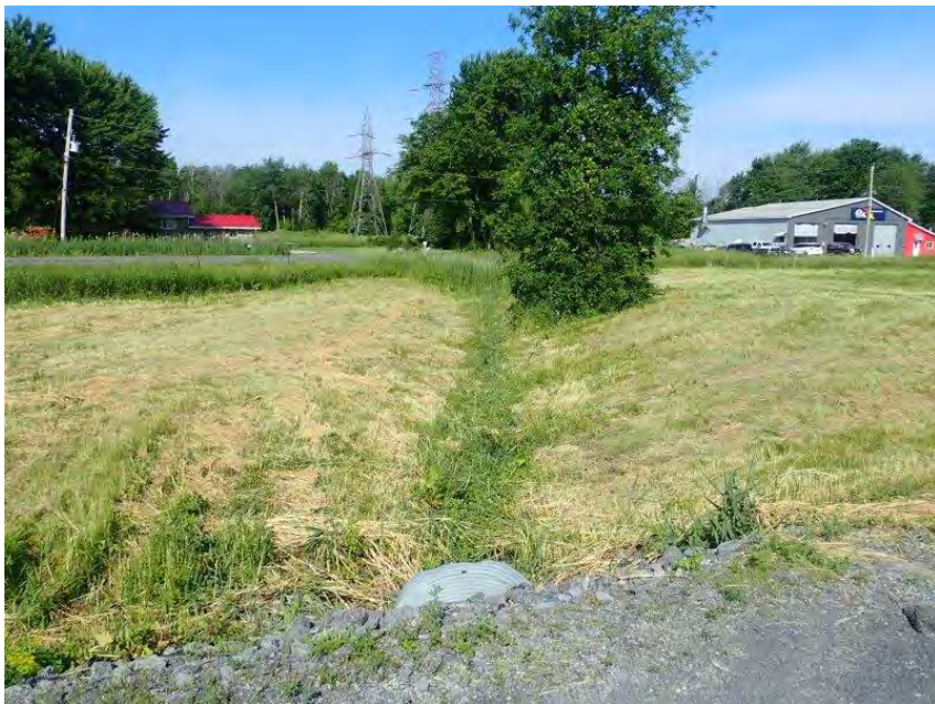
Photo 19. C17 – Power Dam Drive – Overview of the culvert inlet and upstream channel during summer. June 29, 2022
