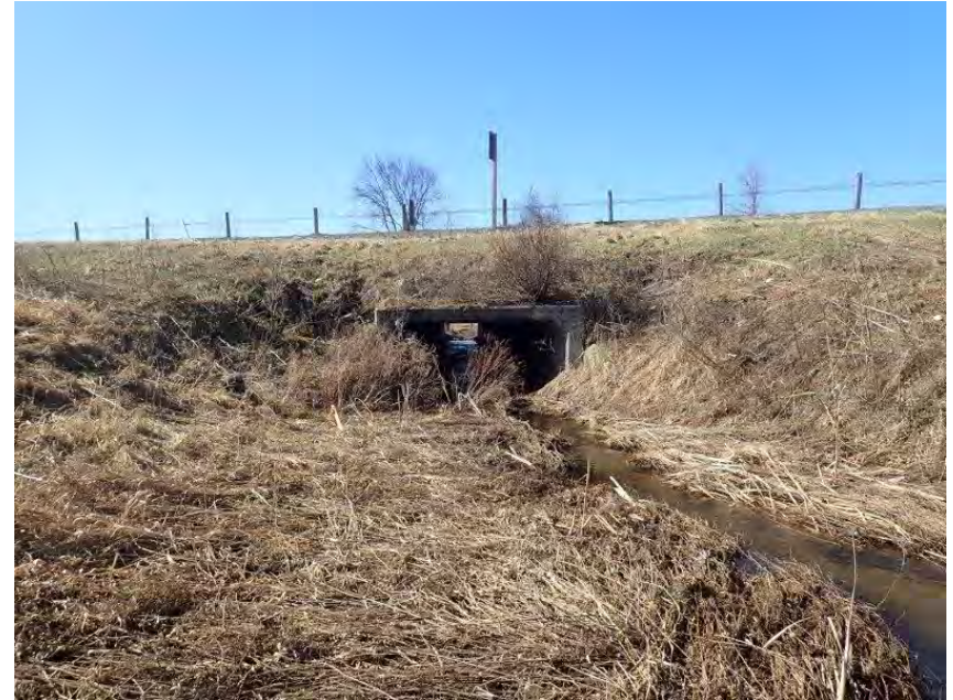
Photo 2. C2 – Highway 401 – View of the culvert inlet and upstream channel flowing to culvert. April 11, 2022
