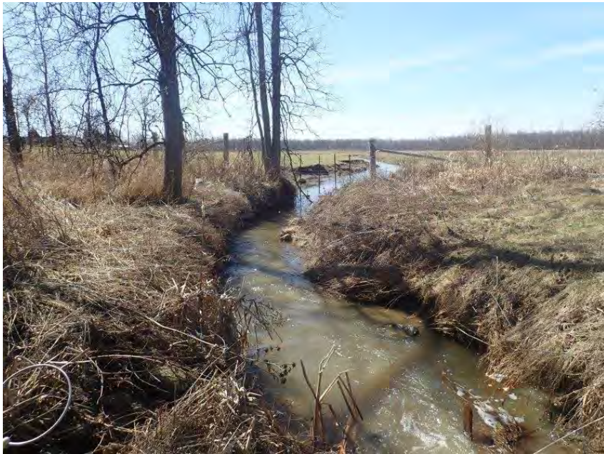
Photo 7. C2 – Highway 401 – Close up view of the downstream channel after culvert outlet. April 11, 2022
