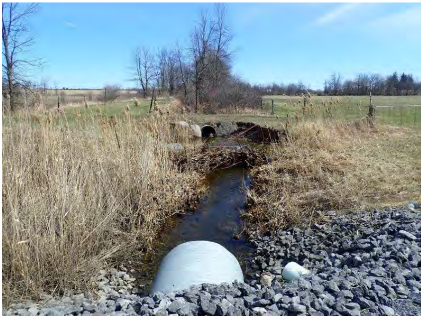
Photo 15. C17 – Power Dam Drive – Overview of the culvert outlet and downstream channel. April 11, 2022
