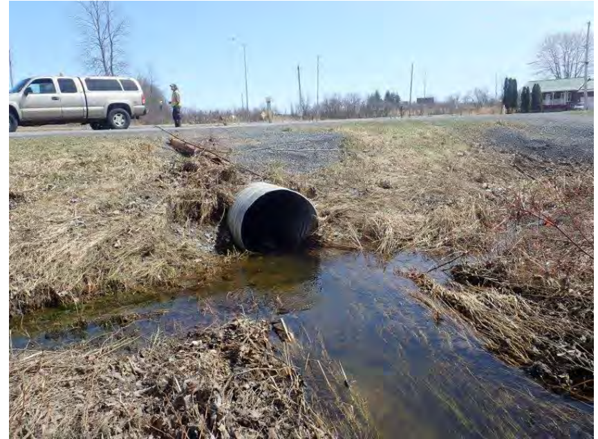
Photo 22. C18 – Atchison Road – View of the culvert inlet. April 11, 2022
