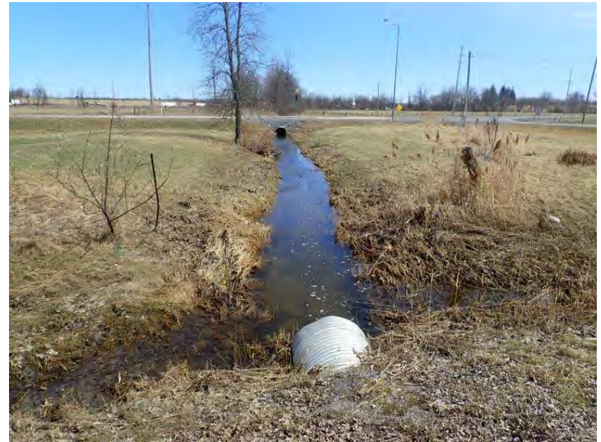
Photo 24. C18 – Atchison Road – Overview of the culvert outlet and downstream channel. April 11, 2022
