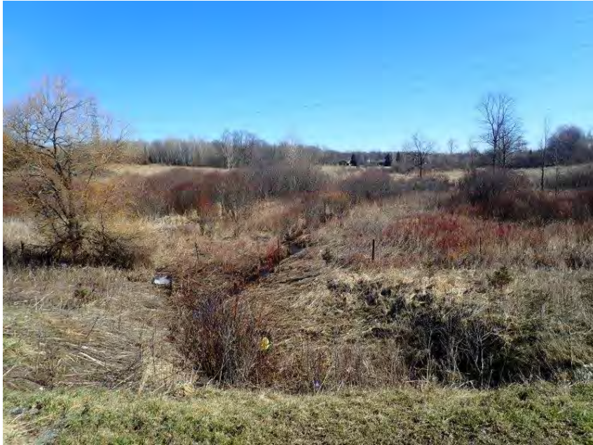
Photo 1. Culvert 2 (C2) – Highway 401 – Overview of the culvert inlet and upstream channel. April 11, 2022
