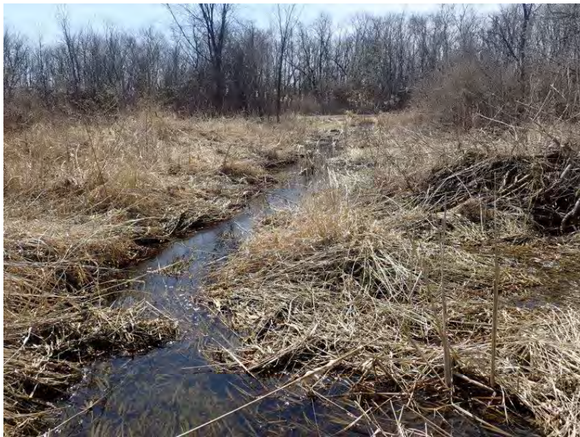
Photo 43. C25 – Highway 401 – View of the downstream channel area. April 11, 2022
