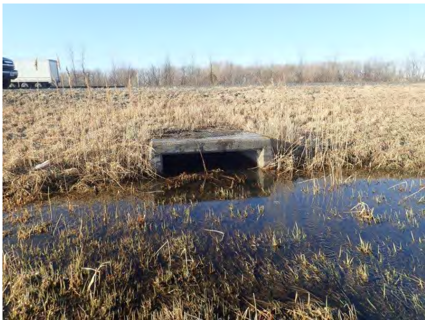
Photo 39. C25 – Highway 401 – View of the culvert inlet with flooded ditchline. April 11, 2022
