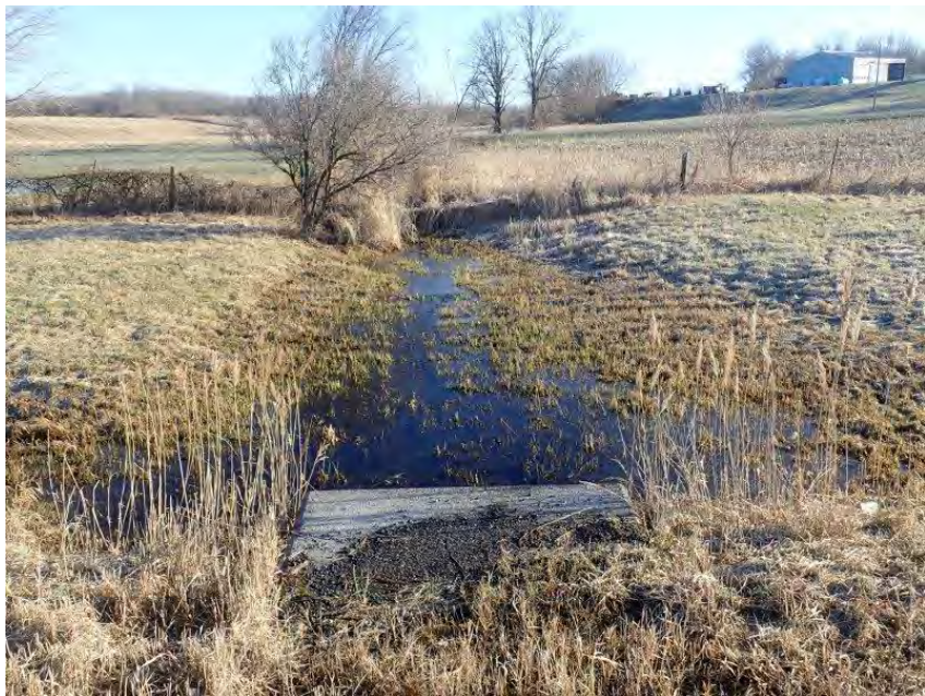
Photo 37. Culvert 25 (C25) – Highway 401 – Overview of the culvert inlet and upstream channel area. April 11, 2022
