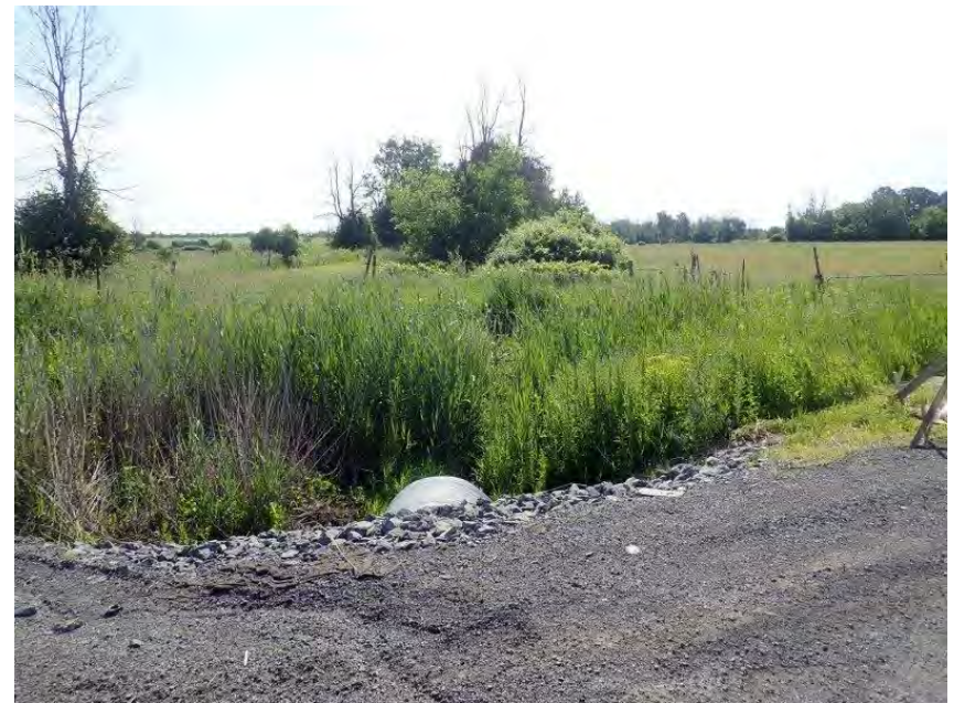
Photo 20. C17 – Power Dam Drive – Overview of the culvert outlet and downstream channel during summer. June 29, 2022
