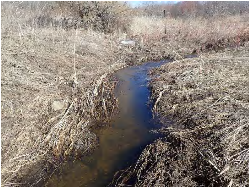
Photo 3. C2 – Highway 401 – View of the channel upstream of the culvert inlet. April 11, 2022
