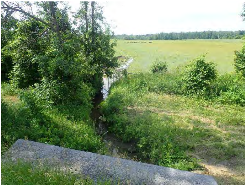
Photo 11. C2 – Highway 401 – Overview of the culvert outlet and downstream channel during summer. June 29, 2022
