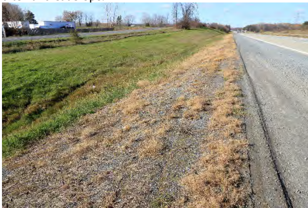
Image 15: West view of the eastbound 401 showing ditch and cut slope.
