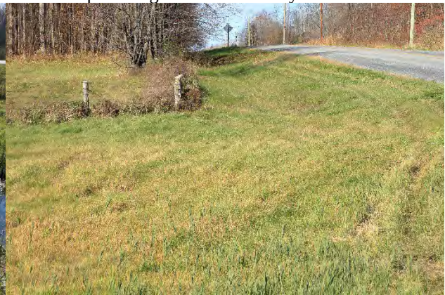
Image 18: North view of the ditch at the corner of the westbound 401 onramp and Power Dam Drive north.
