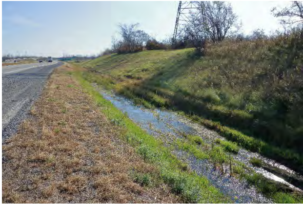
Image 13: East view of the eastbound 401 showing wide ditch and cut slope.
