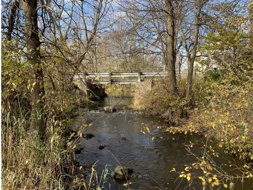
Plate 11: View of the timber beam bridge along Barlow Road over the South Raisin River, looking northwest.
