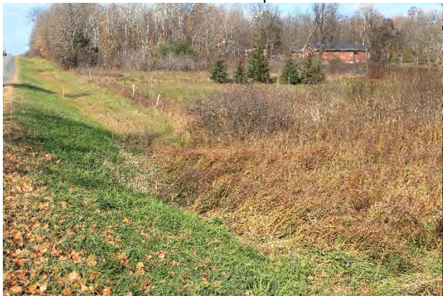
Image 41: North view along the east side of Power Dam Drive with a deep ditch.
