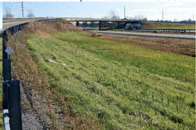
Image 22: East view of the westbound 401 showing wide ditch and filled bridge slope.
