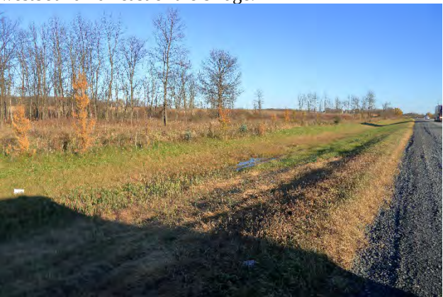
Image 28: East view of the westbound 401 showing wide ditch.
