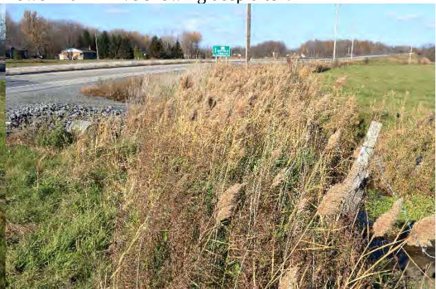
Image 46: North view along the east side of Power Dam Drive showing deep ditch.
