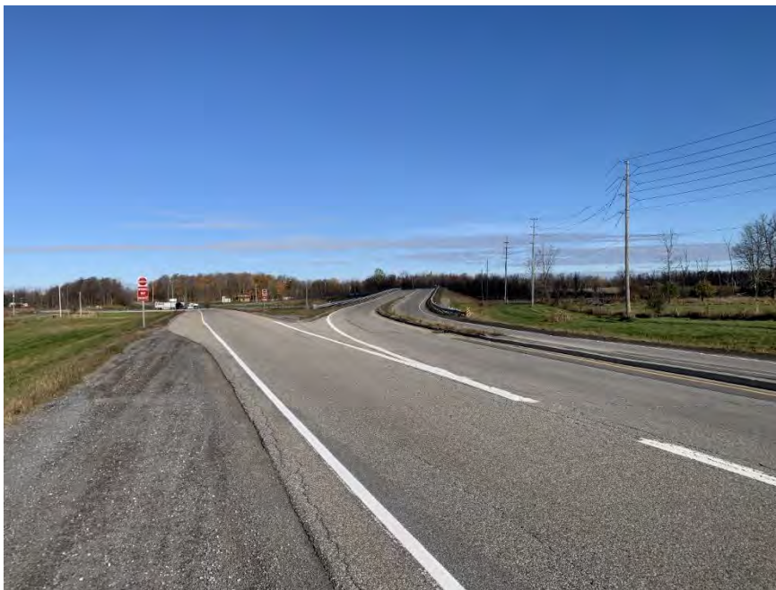
Plate 1: View of the exit to Power Dam Drive and the bridge carrying Power Dam Drive over Highway 401, looking north.
