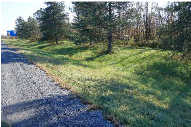
Image 27: East view of the eastbound 401 showing wide ditch and low berm.
