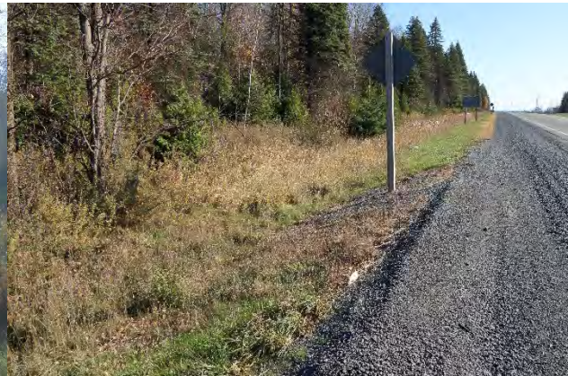
Image 4: East view of the westbound 401 showing wide ditch and cut slope.
