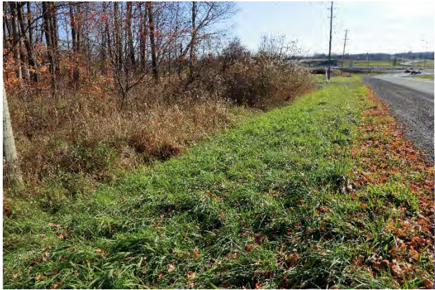
Image 37: South view along the east side of Power Dam Drive with a deep ditch.
