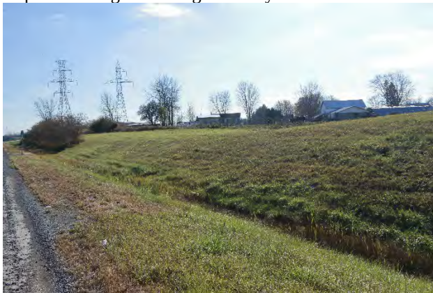
Image 11: East view of the eastbound 401 showing wide ditch and cut slope.
