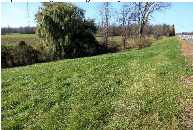
Image 9: West view of the eastbound 401 with a broad slope to the edge of the right-of-way.
