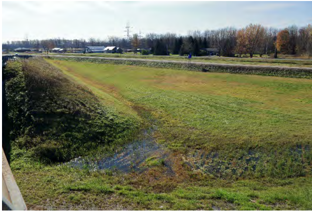
Image 19: South view of the landscaped area between the eastbound 401 off-ramp and bridge.
