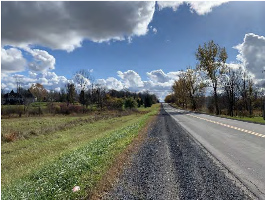
Plate 4: Looking south-southeast along Power Dam Drive from north of the Highway 401 interchange.
