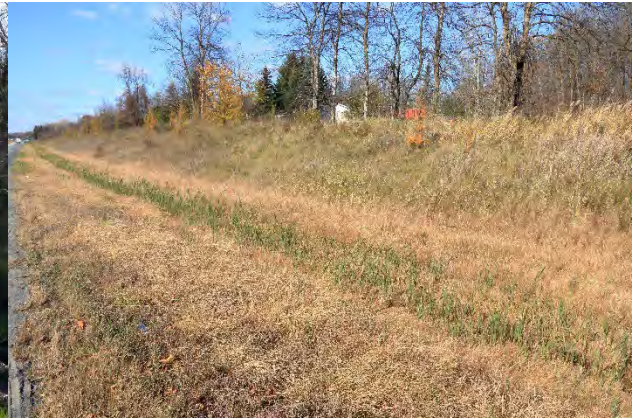
Image 14: West view of the westbound 401 showing ditch and cut slope.
