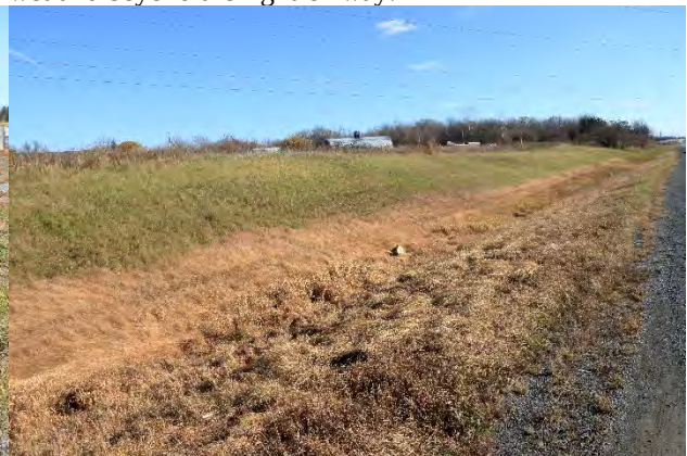
Image 10: East view of the westbound 401 showing wide ditch and cut slope.
