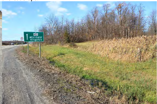
Image 16: West view of the westbound 401 showing ditch and cut slope and agricultural field beyond ROW.
