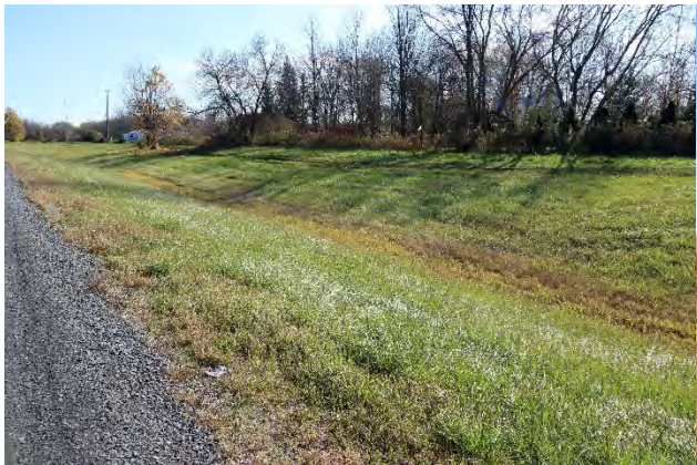
Image 29: East view of the eastbound 401 showing wide ditch and low berm.
