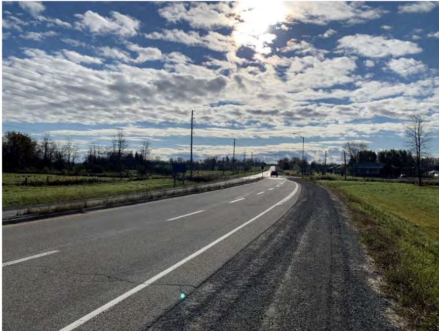
Plate 2: Looking south-southeast along Power Dam Drive from south of the Highway 401 interchange.
