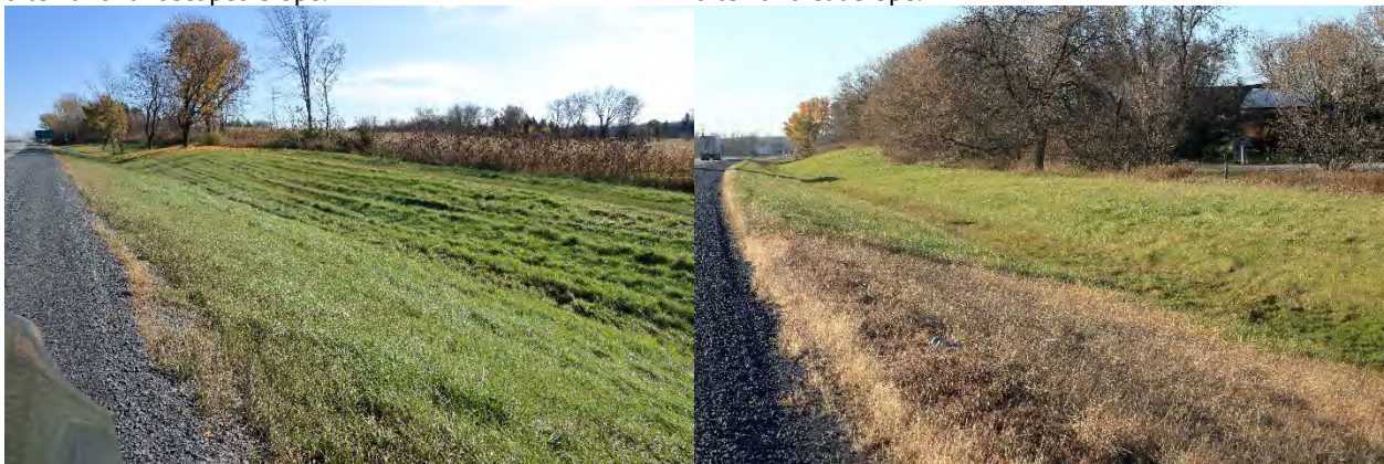
Image 33: East view of the eastbound 401 showing wide ditch and cut slope.
