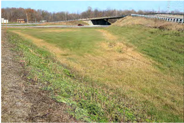
Image 43: North view of the landscaped area between eastbound 401 off-ramp and bridge.
