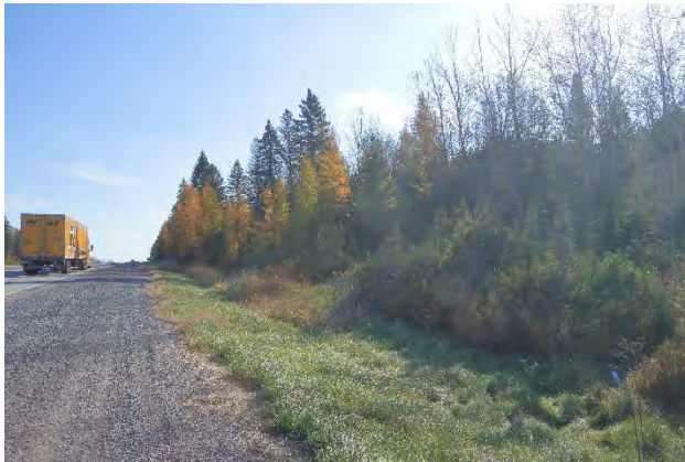
Image 3: East view of the eastbound 401 showing wide ditch and cut slope.
