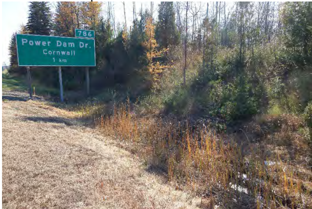
Image 5: East view of the eastbound 401 showing wide ditch and cut slope.
