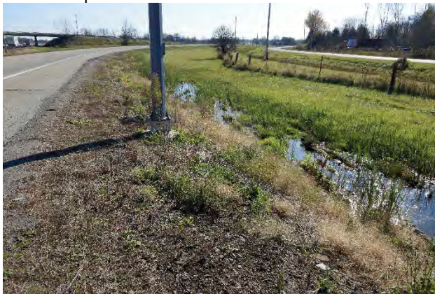
Image 17: East view of the eastbound 401 exit at Power Dam Drive showing wide ditch.
