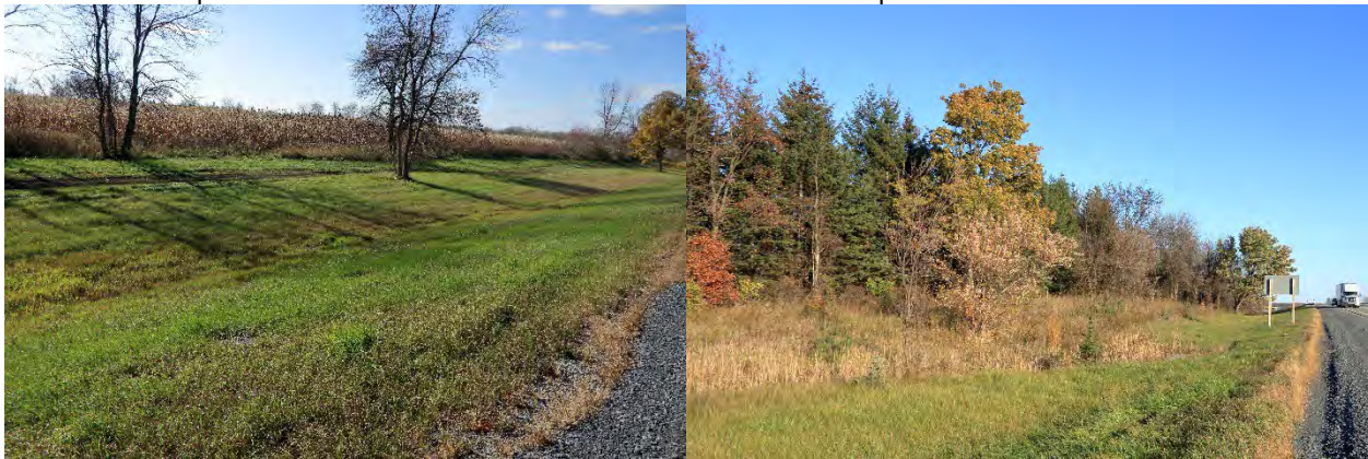
Image 35: West view of the eastbound 401 showing wide ditch and cut slope.
