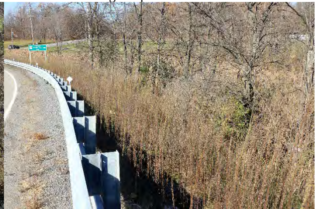
Image 24: West view of slope to the wet area on the north side of Power Dam Drive bridge.
