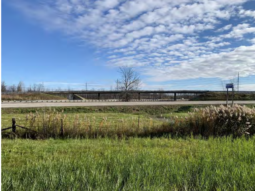
Plate 3: View of the four-span bridge carrying Power Dam Drive over Highway 401 from Atchison Road, looking east.
