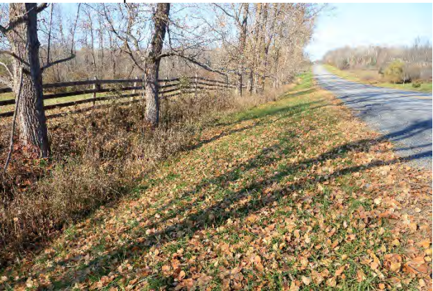
Image 42: North view along the west side of Power Dam Drive with a deep ditch.
