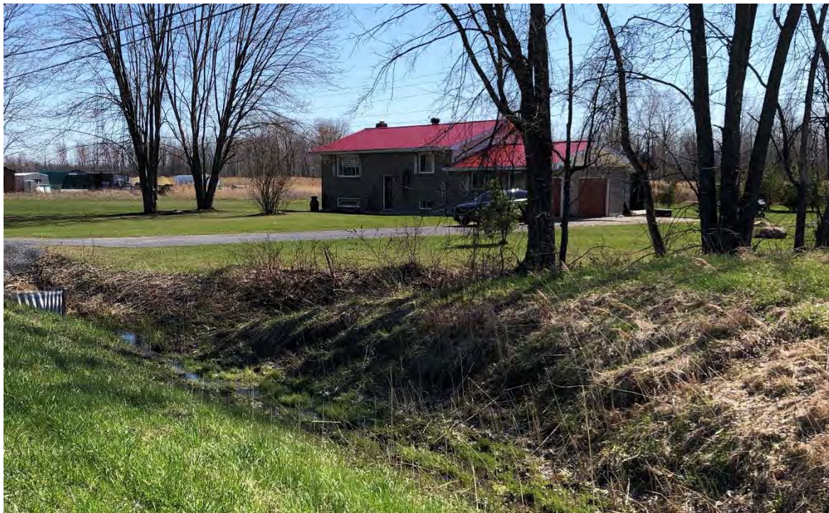
Photo #4 Residential houses and roadside ditches
