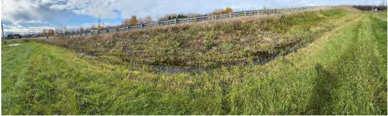
Figure 11: Full ditch along east side of Power Dam Drive embankment, South of Hwy 401
