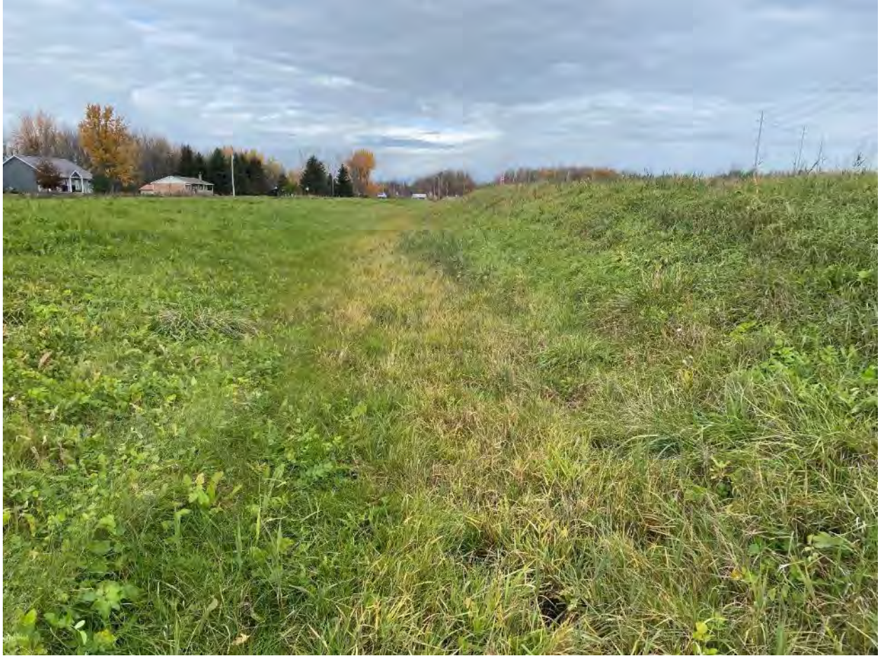
Figure 4: Ditch leading to C17 Culvert under Power Dam Drive
