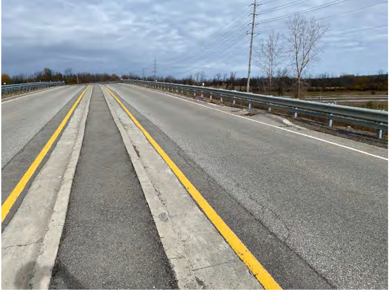
Figure 36: SSC10, C14 - CB inlet and lead; Power Dam Drive Northbound
