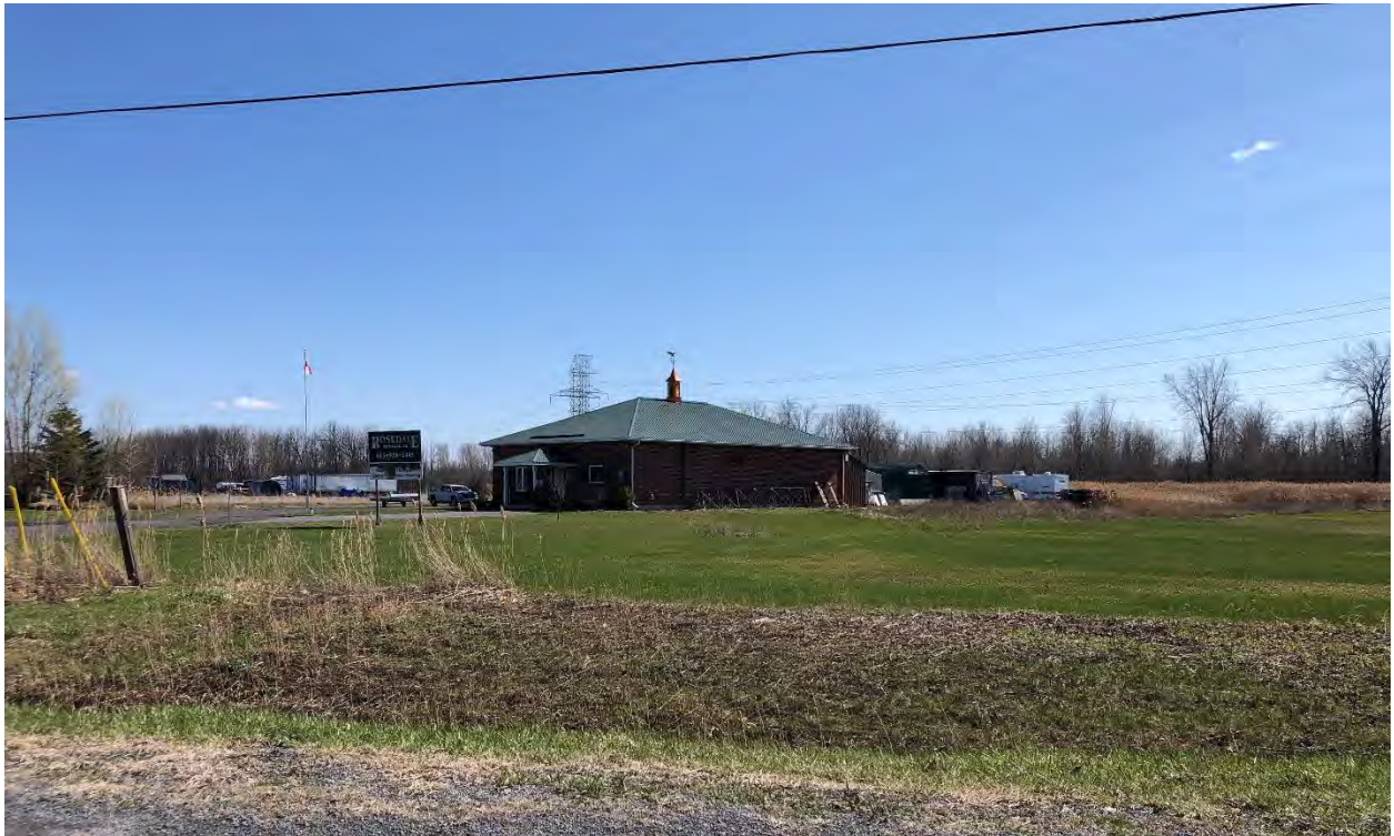
Photo #2 Rosedale Mechanical
