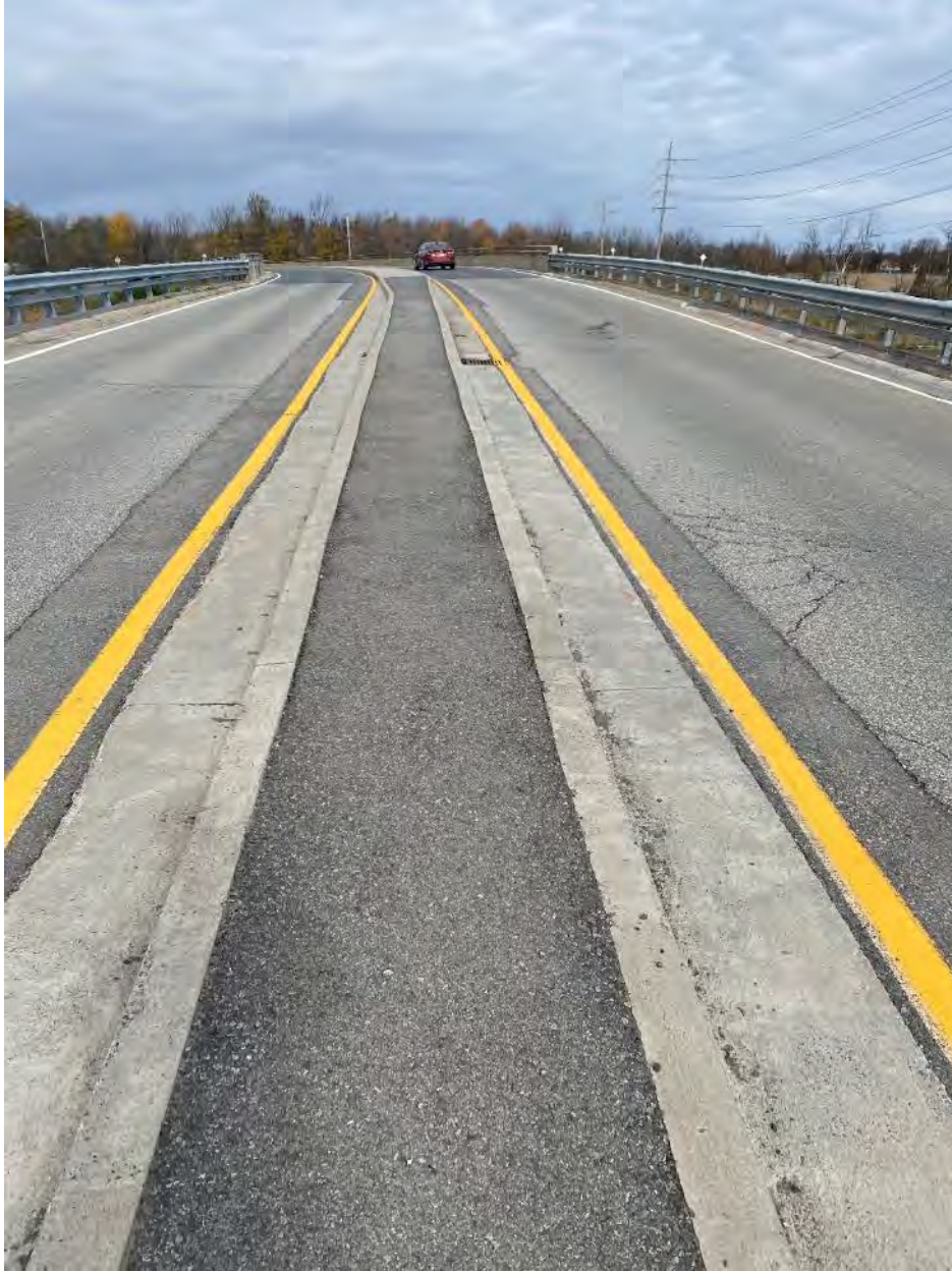
Figure 37: SSC9, C13, CB and Lead Power Dam Drive Northbound
