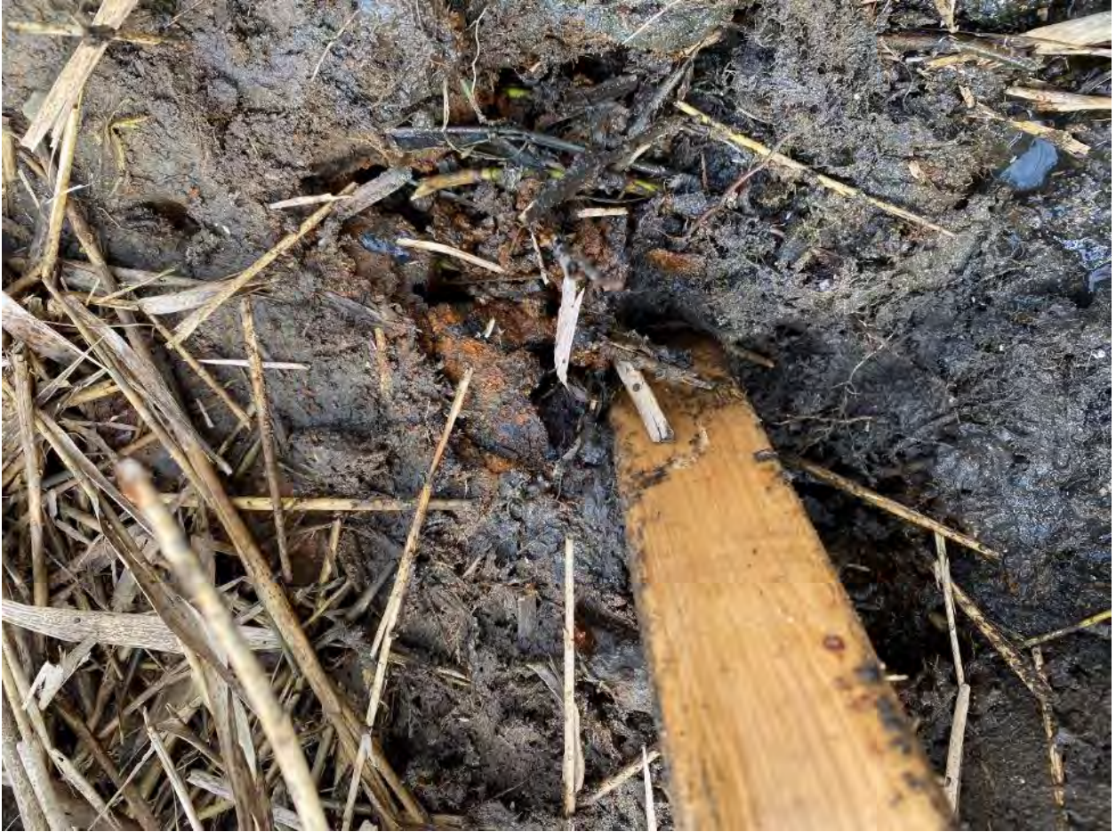
Figure 13: Daylighted CB outlet (SSC10/C14)
