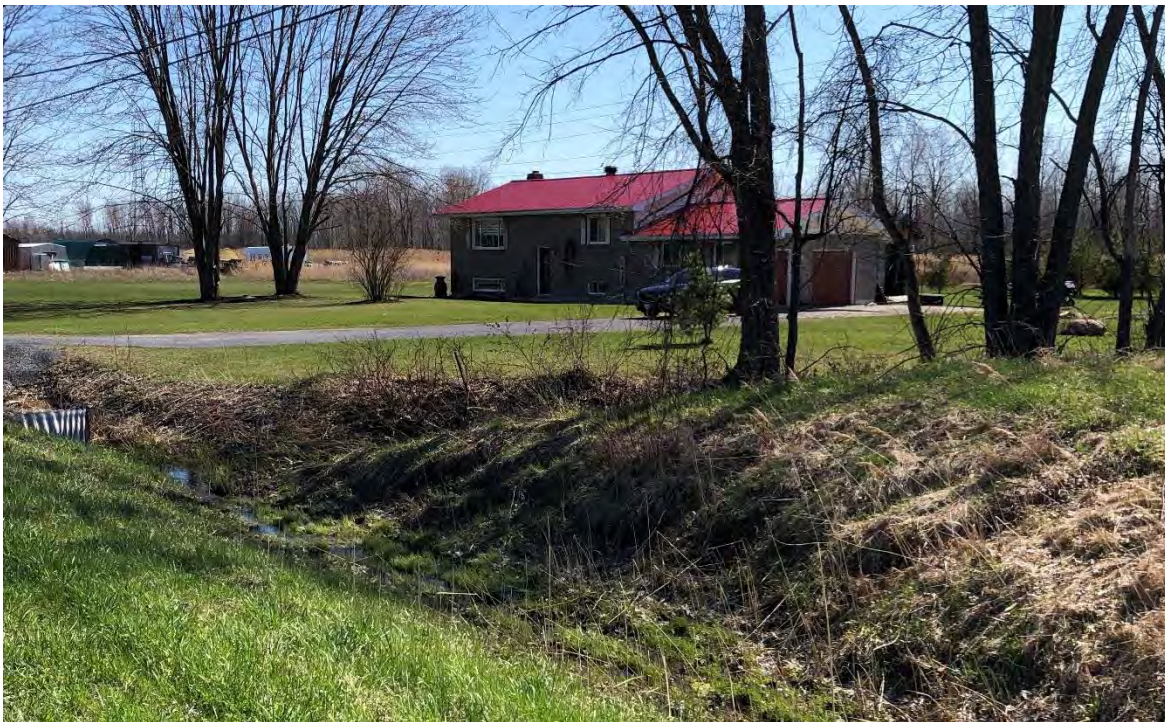
Photo #4 Residential houses and roadside ditches
