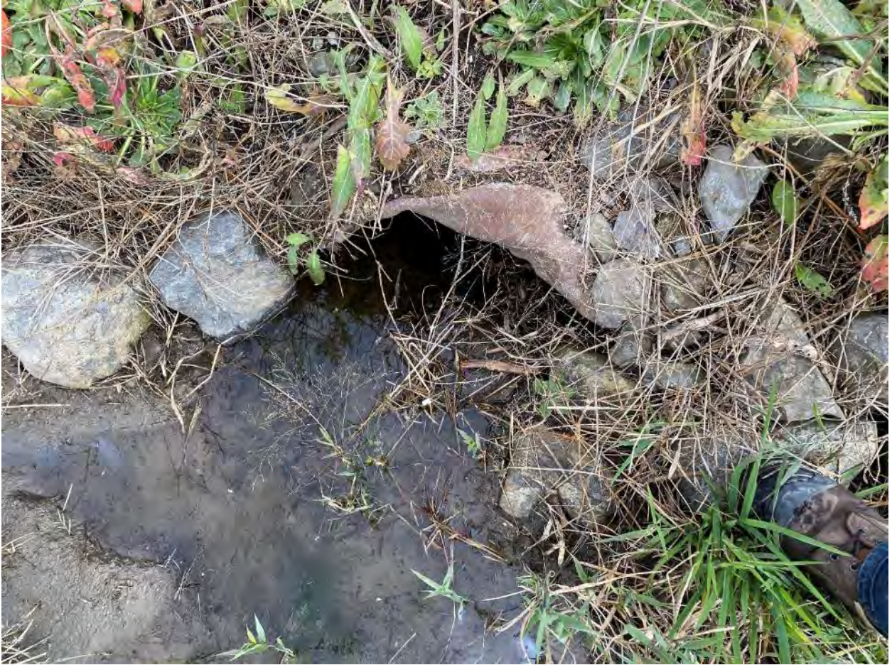
Figure 31: Culvert C7 inlet
