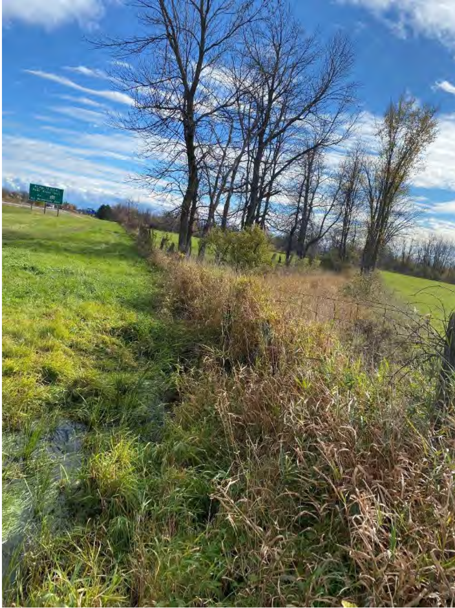
Figure 42: Downstream of C20 leading to municipal drain (ultimate receiver of this drainage area)
