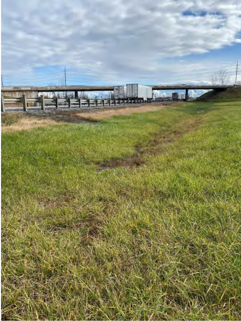
Figure 28: Limited ditch on south side of Hwy 401 from exit ramp to C5
