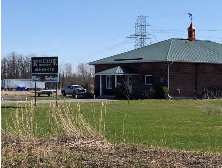
Photo #1 Rosedale Mechanical
