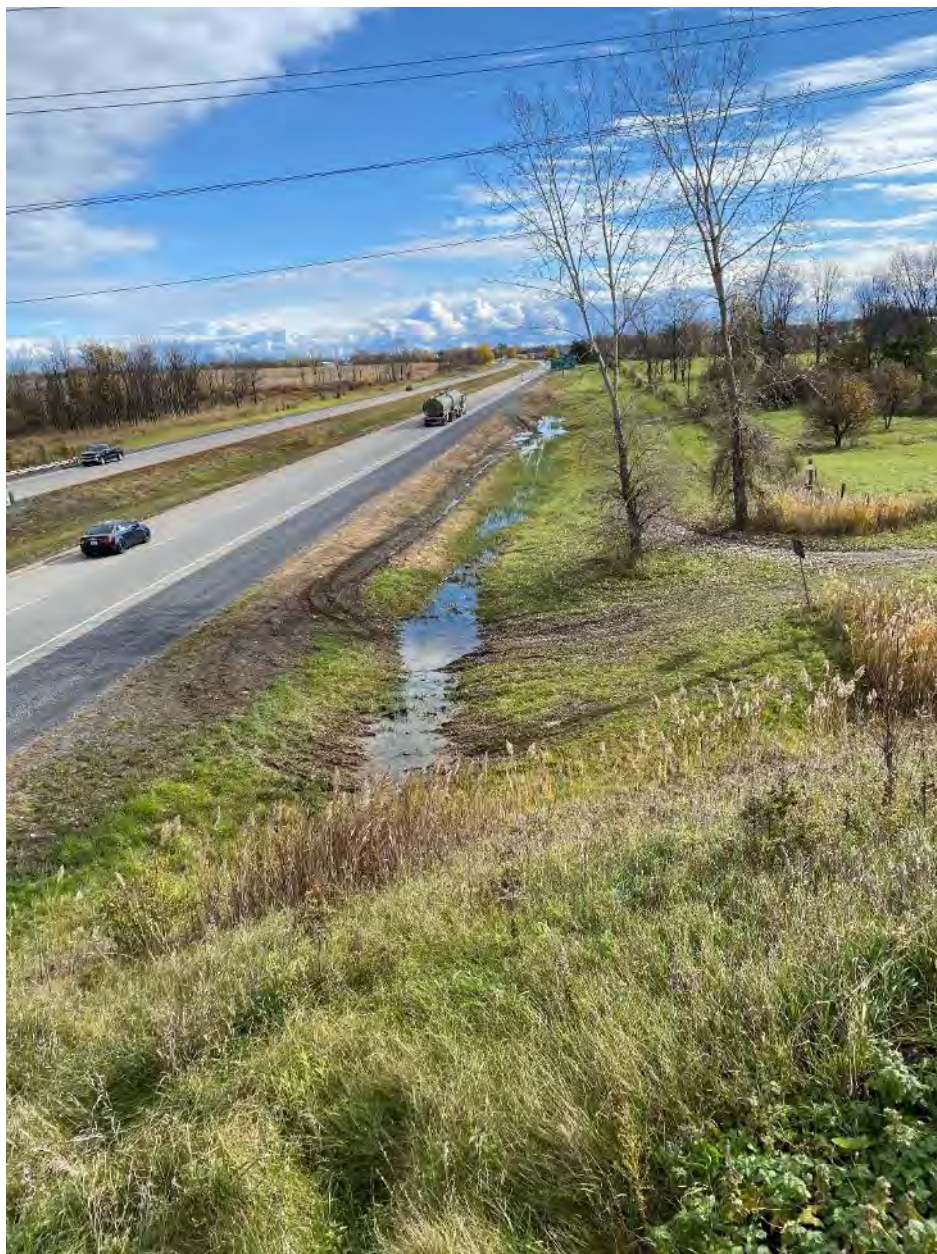
Figure 39: Drainage area East of Power Dam Drive, South of Hwy 401
