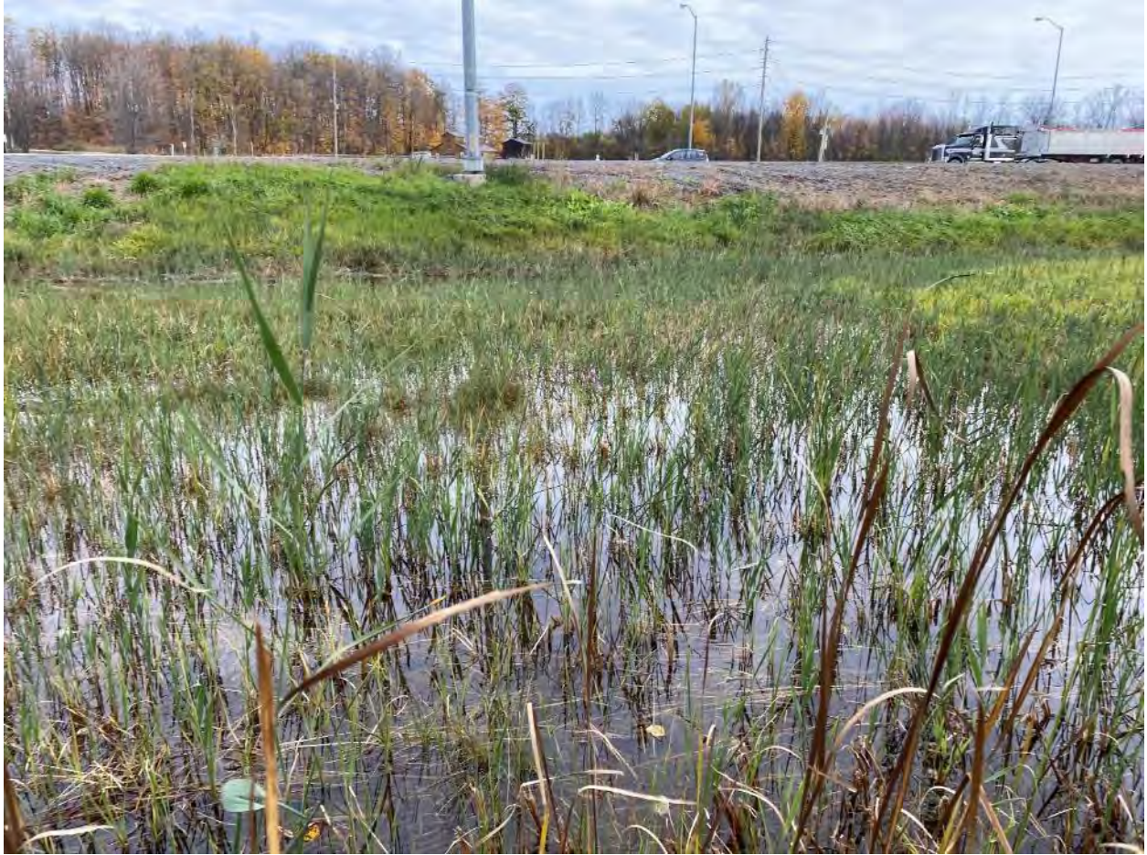
Figure 1: Ponding south of Hwy 401 near Culvert C7
