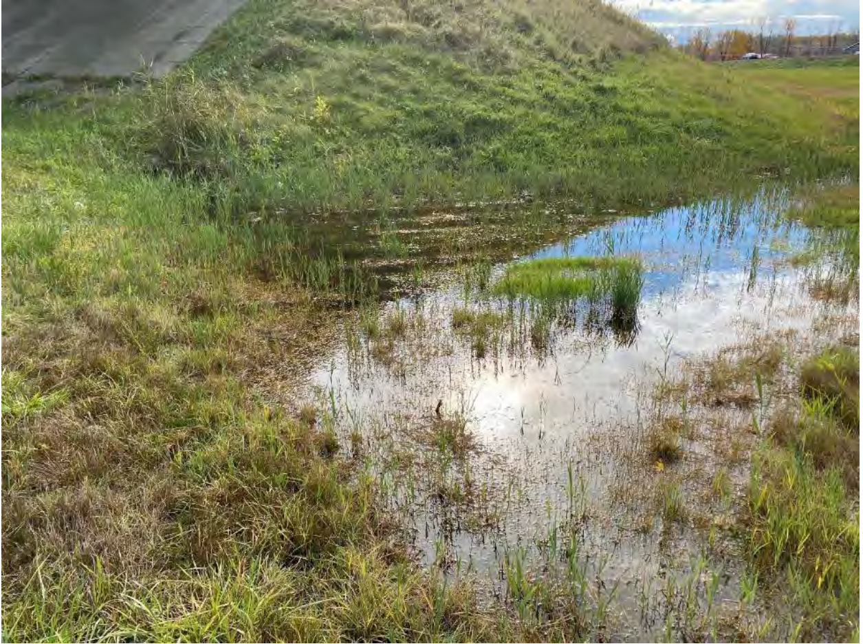
Figure 23: Ponding upstream of C8 (S-W of Hwy 401 and Power Dam Dr)
