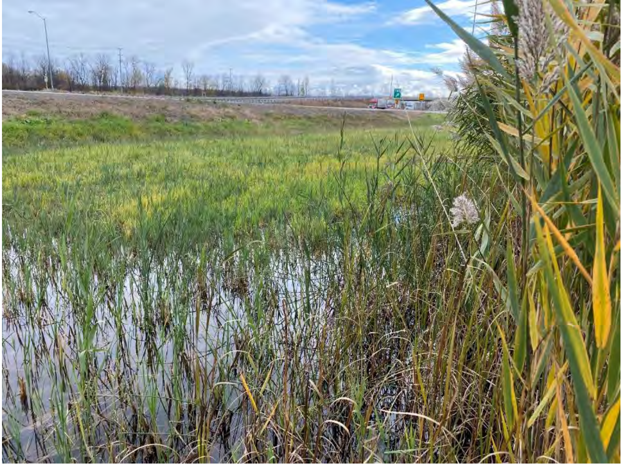
Figure 2: Ponding south of Hwy 401 near Culvert C7
