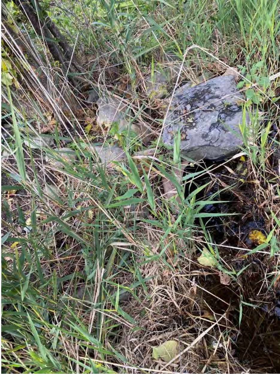
Figure 33: Culvert C7 Outlet
