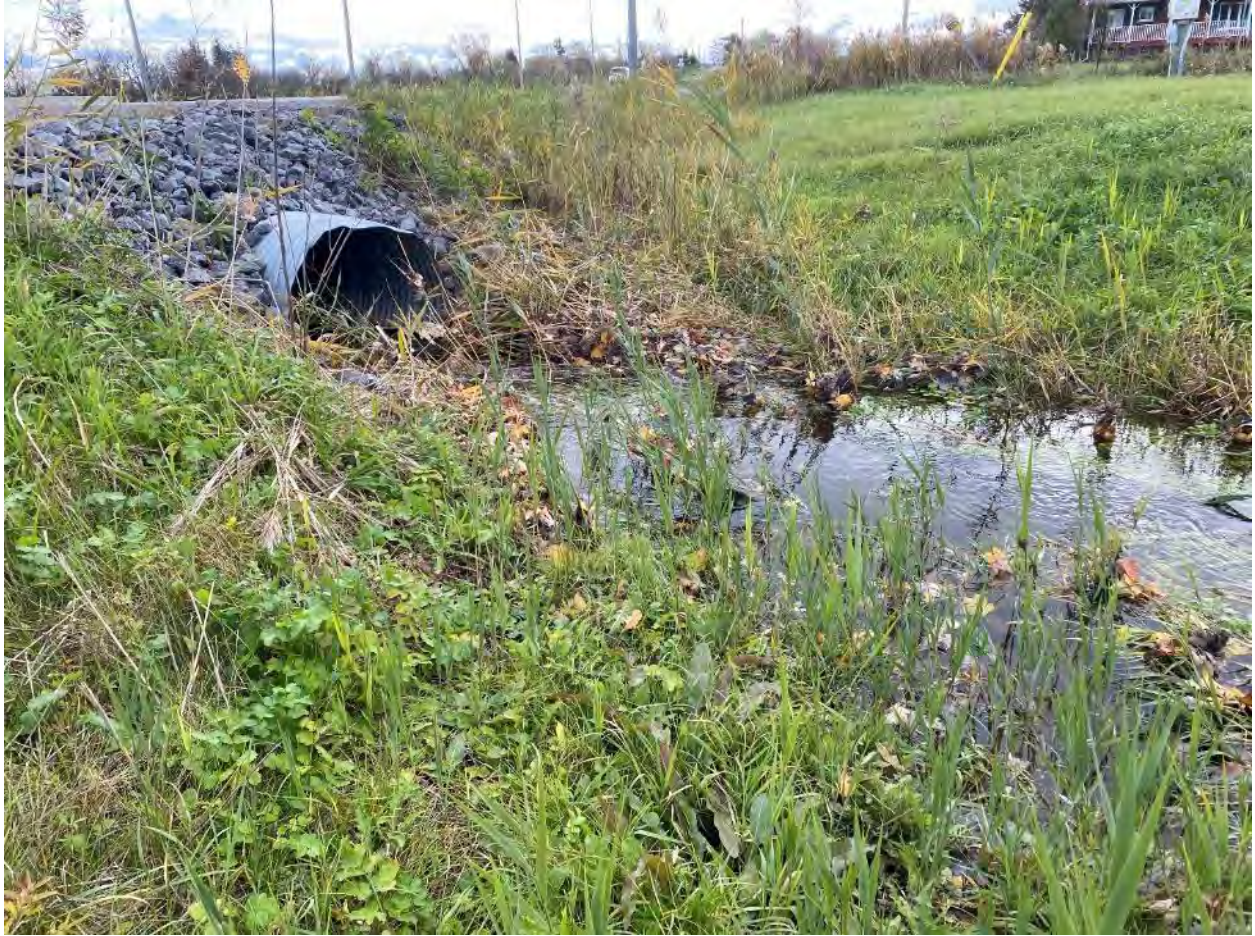
Figure 5: Inlet of Culvert C17 under Power Dam Drive, 1200 mm, good condition, 350 mm water depth
