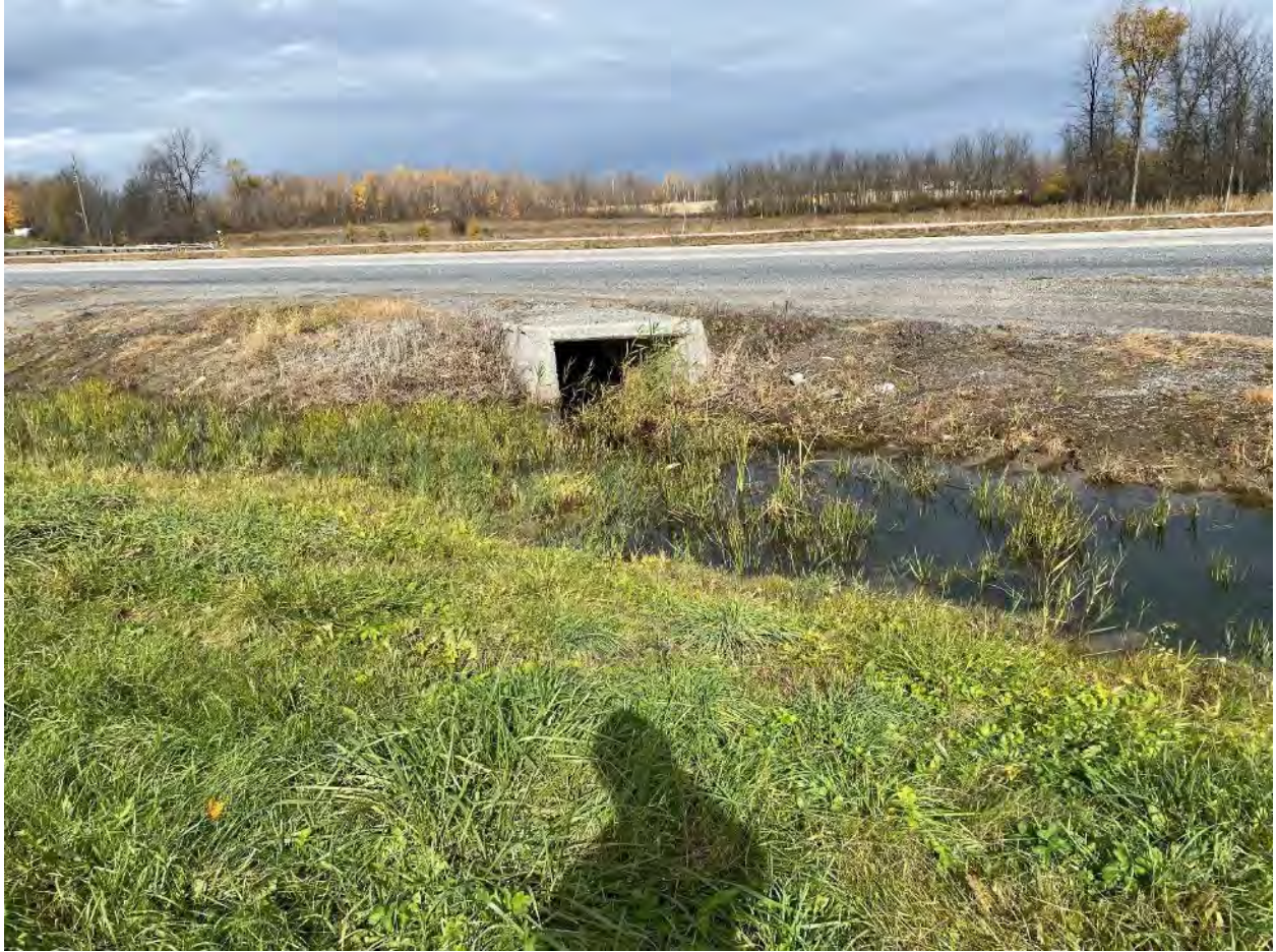
Figure 40: C19-C20 carrying flows across Hwy 401 (south side)
